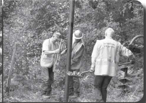
Tamping The Posts In Place With Rock.
