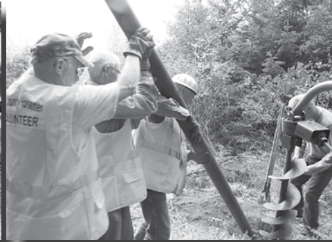
Lifting the 12 foot steel post in place.
