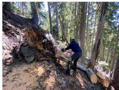
Last cut project of the entire trip. A bit of a fun jackstraw puzzle (piled on top of each other, loose rootball, snag in the way, and a steep hillside gave it just enough challenge to be fun).
